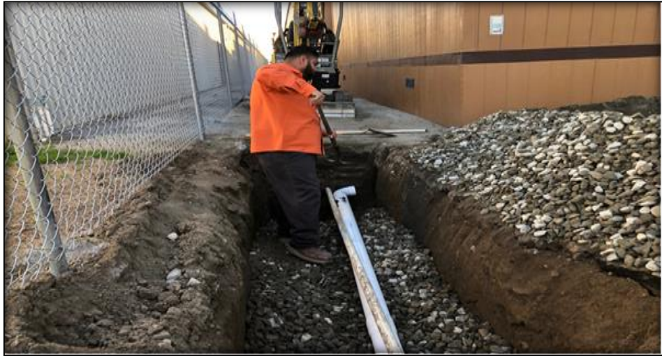
Crews made drainage improvements to City Yard
