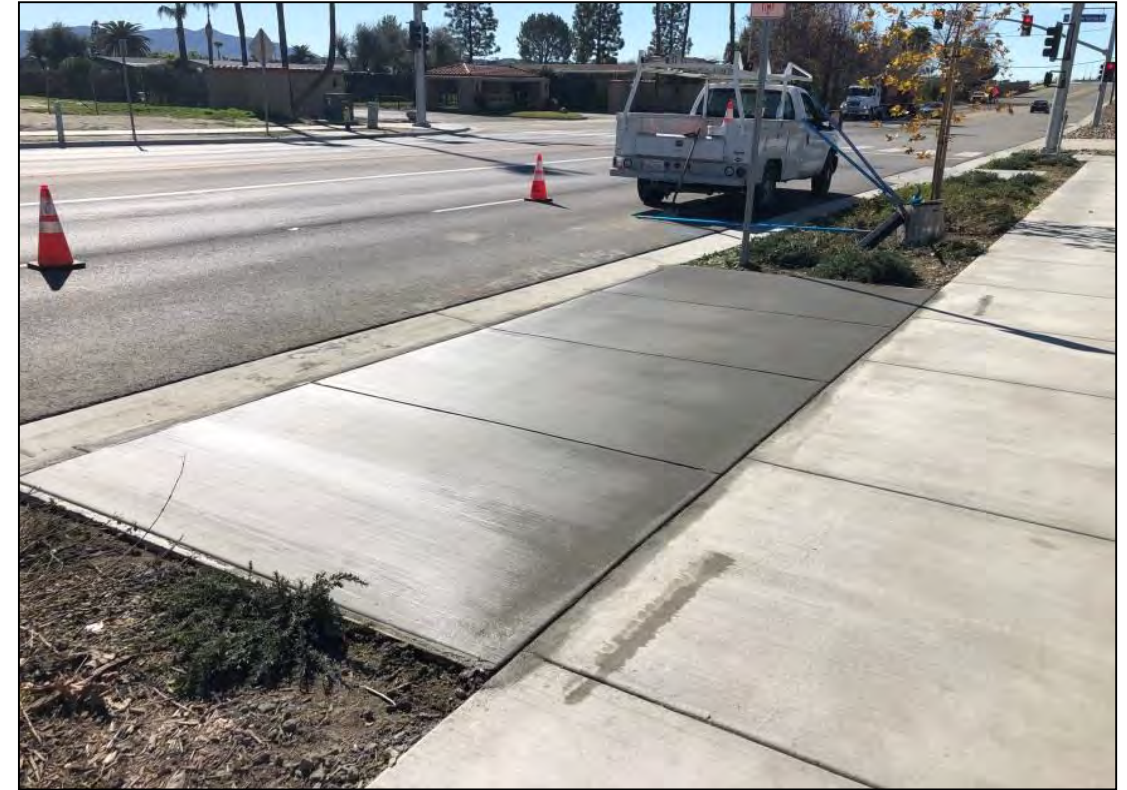
Staff installed an 8X20 concrete slab for a future bus stop on Lake Park Drive
