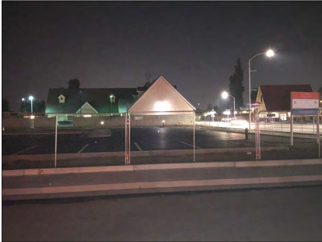
Improved LED lighting installed on the north exterior of City Hall
