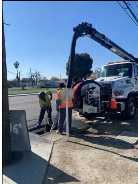
Vault vacuuming at State Street and Cottonwood Avenue
