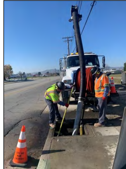
Vault vacuuming at State Street and Cottonwood Avenue
