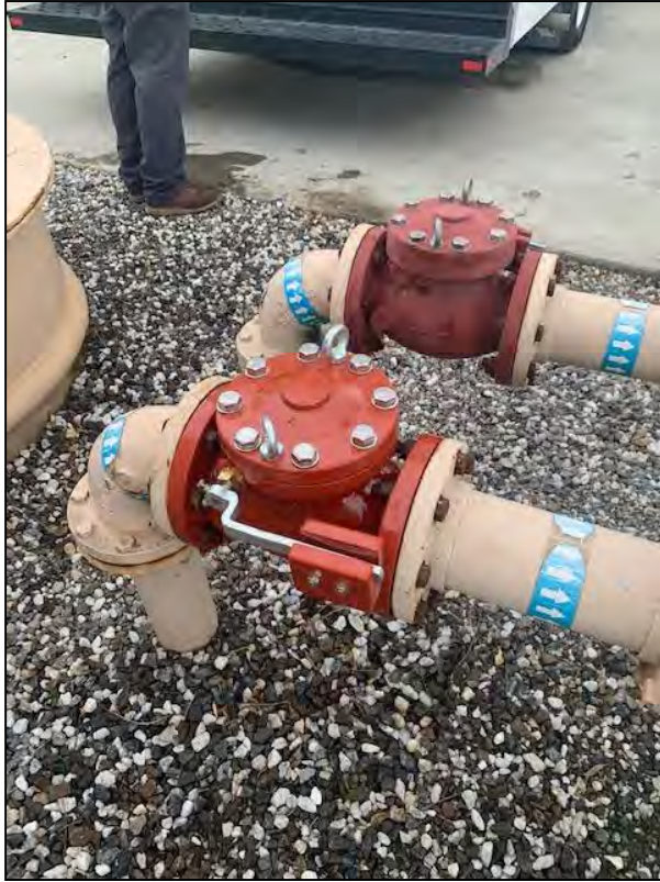
Check valve replacement at Cottonwood Lift Station
