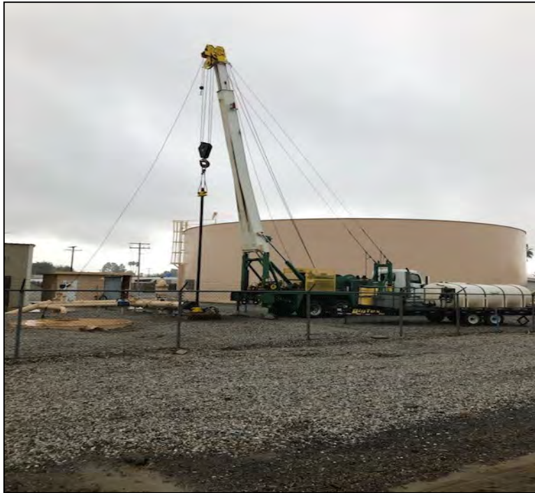
Bath Well pump testing using 1200 HP engine
