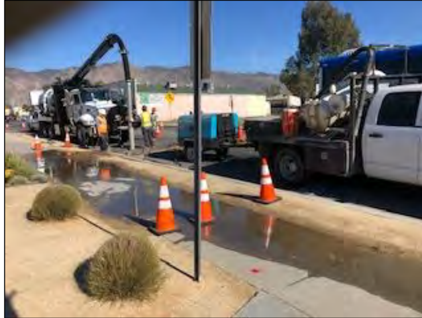
Pipe repair on San Jacinto Avenue
