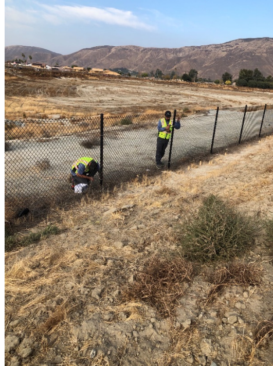
Re-Securing the fence at the Lyon Avenue Basin
