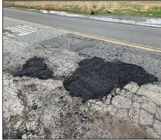
Temporary asphalt repair on Ramona Boulevard near Sanderson
