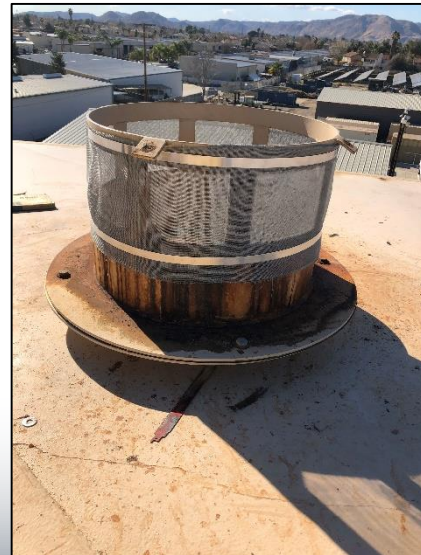
Grand Tank Maintenance - Replacing the steel screen with a finer stainless steel screen
