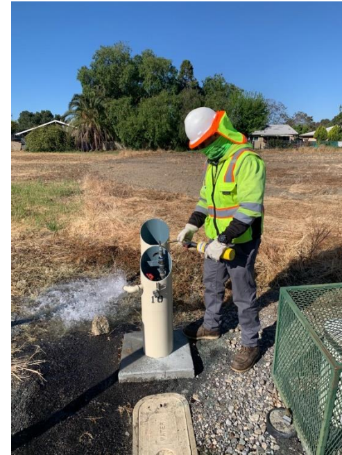
Production Crew preparing to take water quality samples from the sample station on Ramona Boulevard
