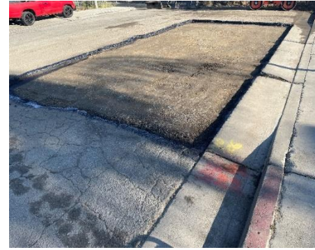
Grind and Overlay – North end of Buena Vista
