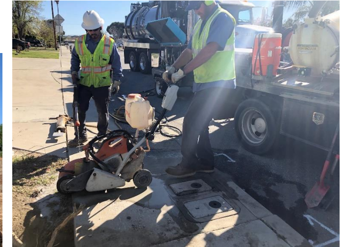
Construction Crew prepares to make repairs to a service line leak
