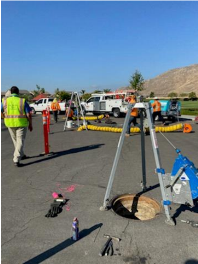
Contractor and Wastewater crews removed sewer blockage left by the original contractor that caused high sewer flow levels on Cherry Laurel Lane in the Tamarisk subdivision
