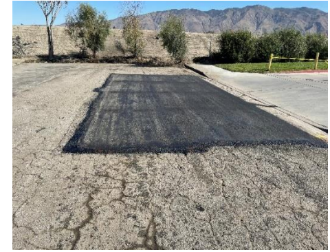
Grind and Overlay – North end of Buena Vista
