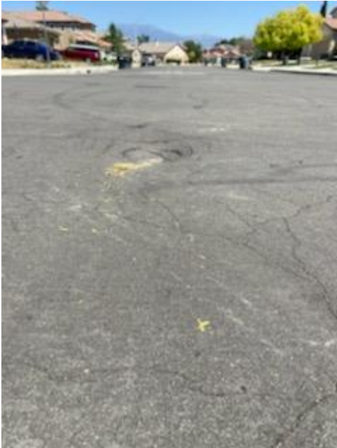
Waste Water, Storm Water and Street Crews filled and repaired a sink hole in the Meadowbrook I subdivision on Grassy Meadows Drive and Sweet Clover Loop
