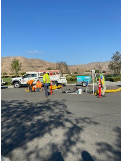
Contractor and Wastewater crews removed sewer blockage left by the original contractor that caused high sewer flow levels on Cherry Laurel Lane in the Tamarisk subdivision
