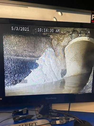
Contractor and Wastewater crews removed sewer blockage left by the original contractor that caused high sewer flow levels on Cherry Laurel Lane in the Tamarisk subdivision
