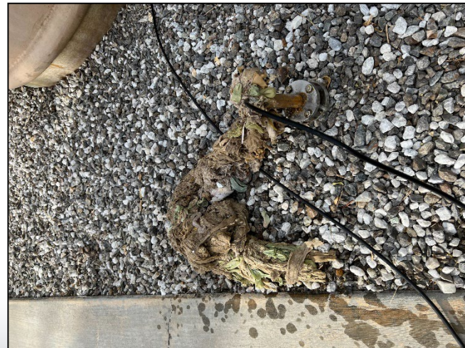
Cottonwood Lift Station clean out
