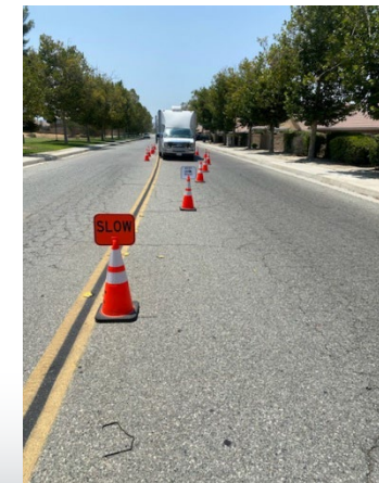
Traffic Control setup while videoing
