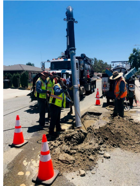
Waste Water assists with a deep service line leak on Salam Place
