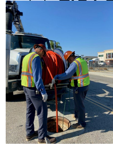
Cleaning the Line on State Street
