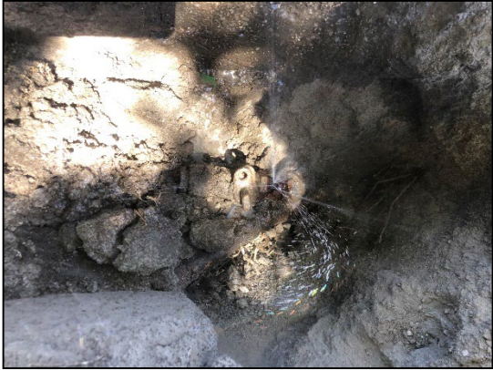
Curb stop replacement at 646 N. Brinton
