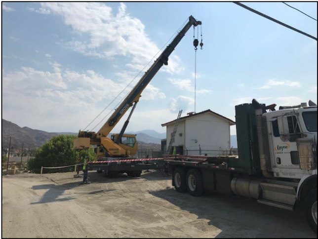
Preparing to remove the roof of the well house
