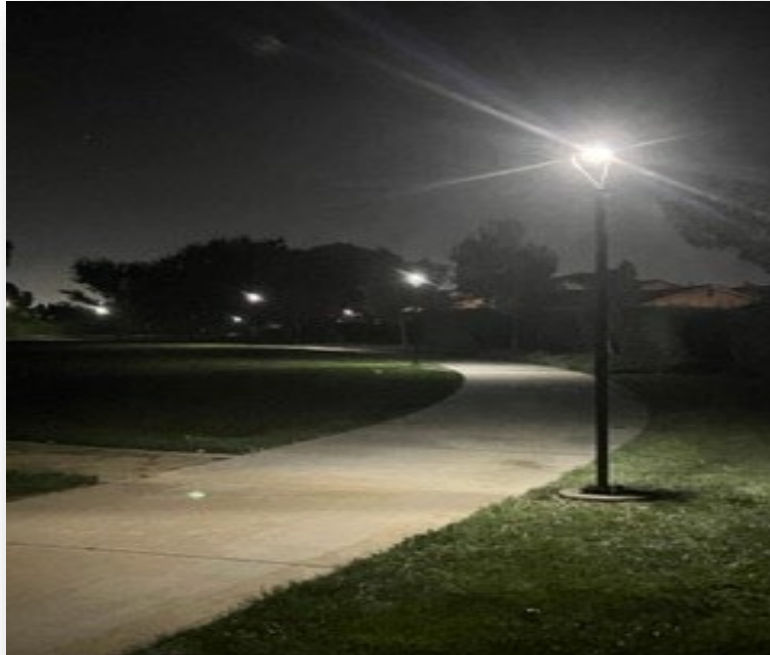
LED Solar Lights installed in Zone 11
