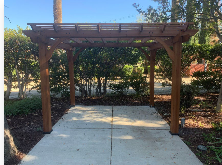
New pergola built and installed at Estudillo Mansion
