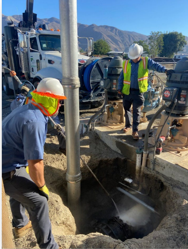
Replacement of 12" valve at Bath Booster
