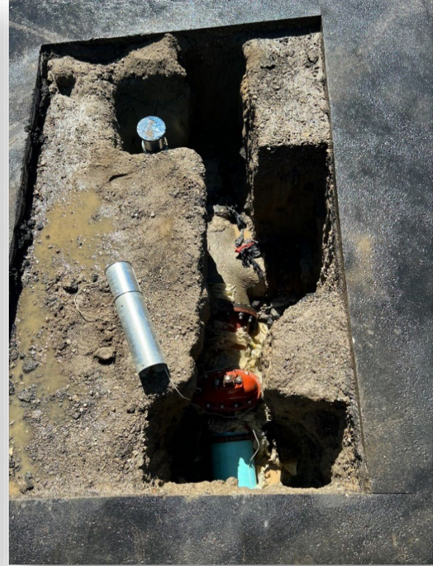
Exploratory potholing at Bath Well and Camino Los Banos for Bath Well Treatment Plant replacement
