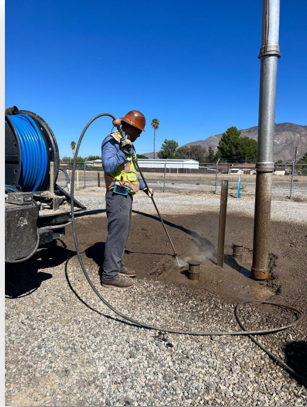
Exploratory potholing at Bath Well and Camino Los Banos for Bath Well Treatment Plant replacement
