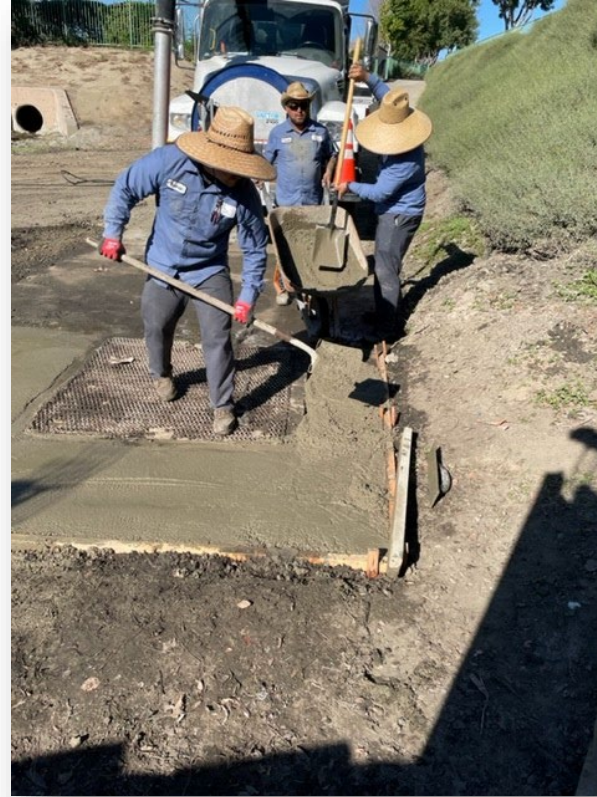
Zone 8 installation of pump vault inlet barrier
