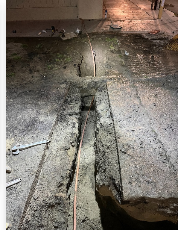
Installation of new copper water service at 210 E Main
