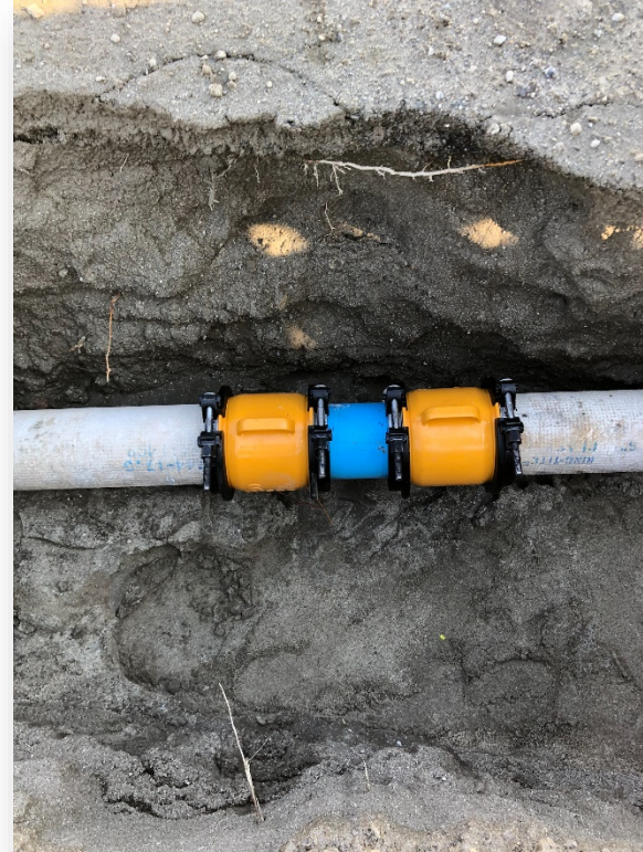
6" water main repair on Alessandro
