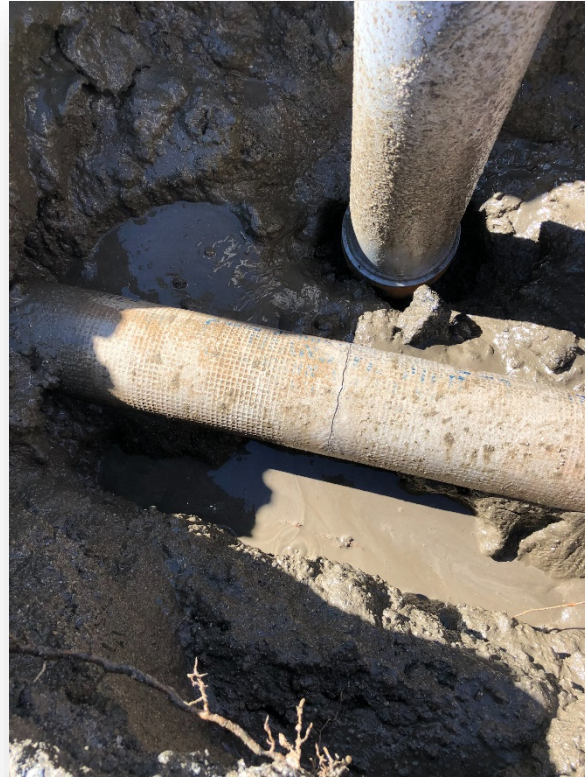
6" water main repair on Alessandro
