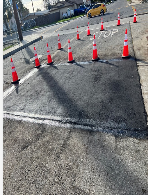
Repaired sinkhole on Shaver and Hewitt
