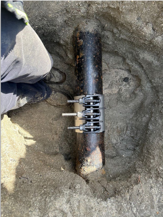
Water Leak Repair on Alessandro
