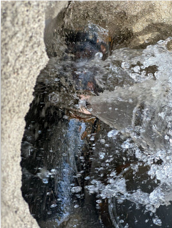
Water Leak Repair on Alessandro
