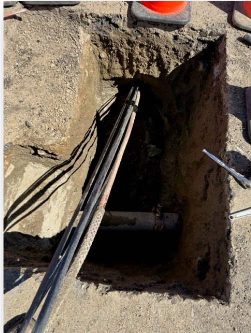
Repaired Water leak repair on Marcy way
