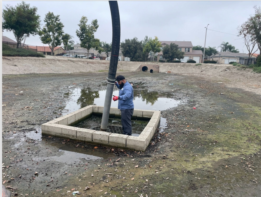
Sediment removal at Lyon Basin
