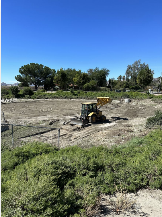
Sediment removal at Lyon Basin
