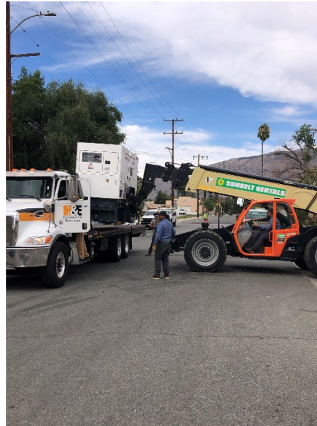
Removal & installation of Police Department's new backup generator
