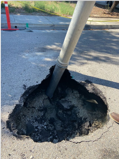
Repair of sinkhole on sewer lateral on Sagecrest Drive
