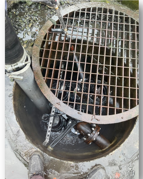
Cleaned Sagecrest pump vaults
