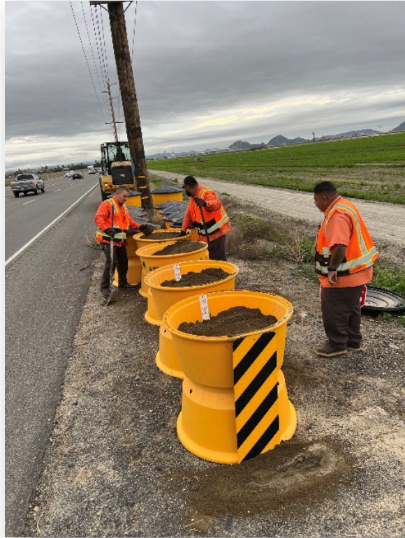
Recovered fallen crash barrels caused by heavy winds and rainfall
