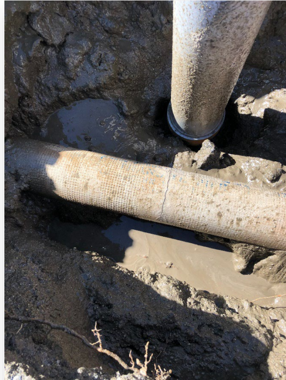
6" water main repair on Alessandro
