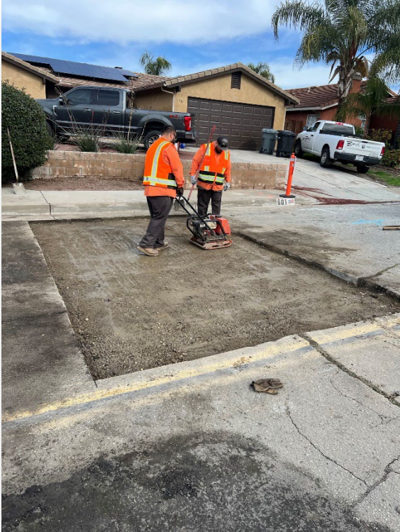
Repaired sinkhole on Shaver and Hewitt
