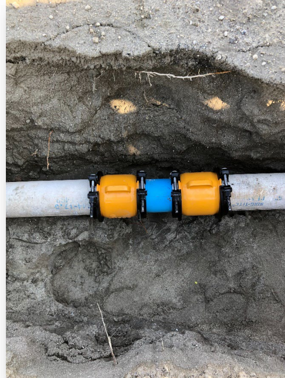
6" water main repair on Alessandro
