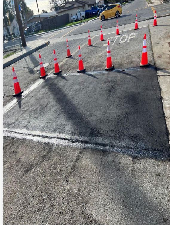
Repaired sinkhole on Shaver and Hewitt
