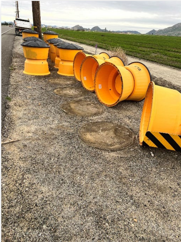
Recovered fallen crash barrels caused by heavy winds and rainfall
