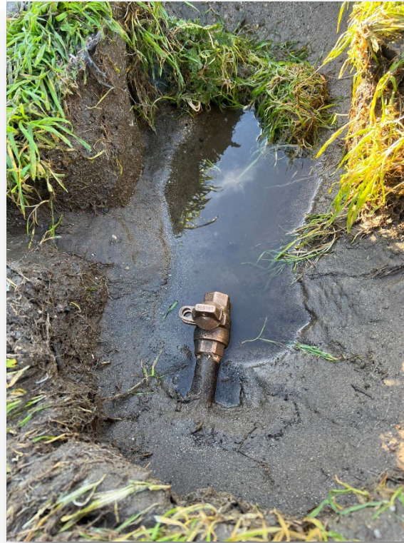
Replacement of broken angle stop on 3 rd Street
