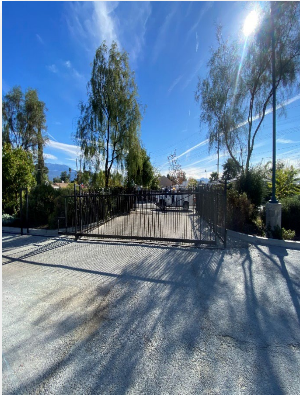
Installation of the Mansion's new electrical gate on Ash Street
